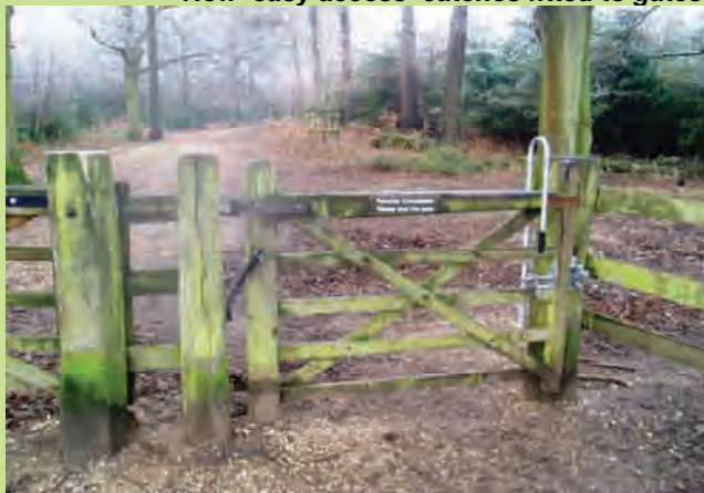
New 'easy access' catches fitted to gates
