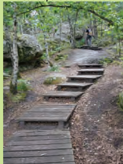
Raised steps to combat erosion
